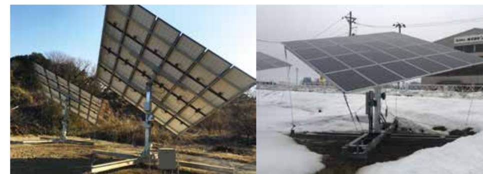
H-Beam Base H 型鋼基樁
